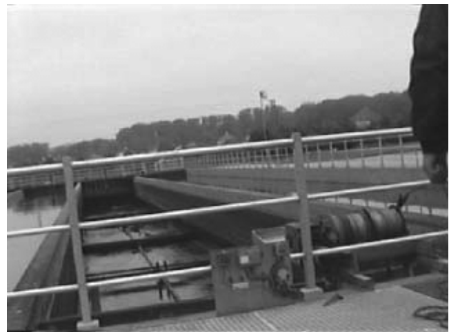
Figure 1: Blacksmith fixing a broken wire in a clarifier tank
