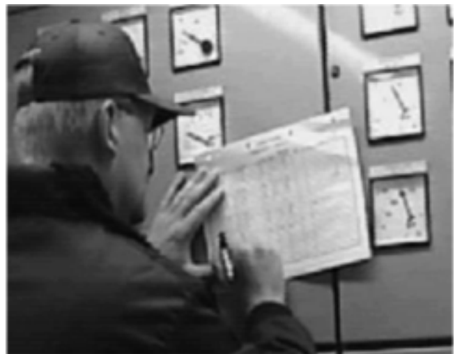
Figure 5: Wastewater operator reading the gas meters
