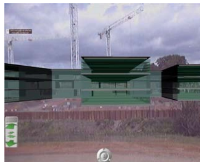
Figure 3: Shows the result of the initial registration using corresponding lines for orientation recovery and manual recovery of the position.
