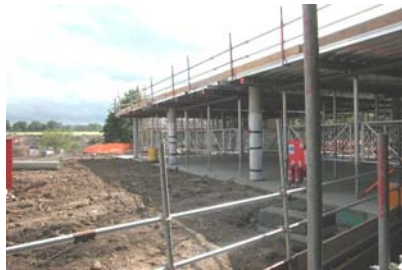
Figure 4: Courtyard building site.
